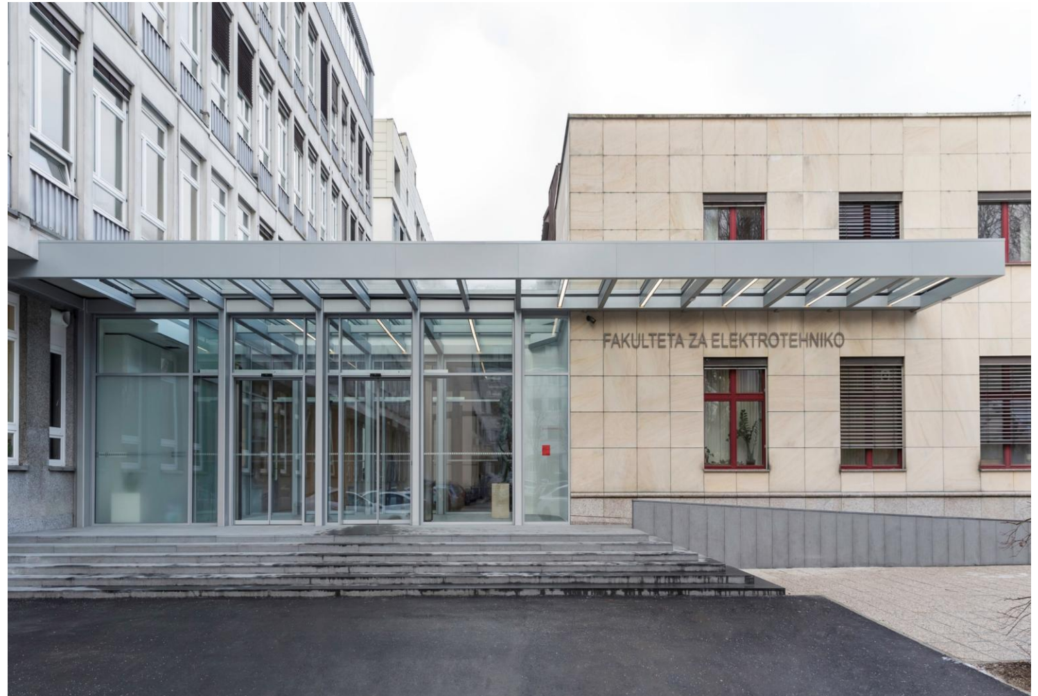
Faculty of Electrical Engineering, Tržaška cesta 25, 1000 Ljubljana
